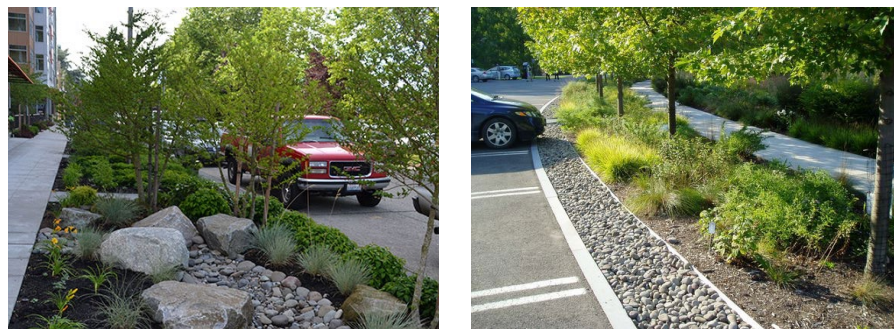
Examples of LID stormwater facilities, which can serve double-duty by replacing lawn park strips with waterwise planting to conserve water while filtering stormwater runoff
