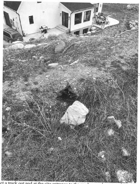
Note: in the rare event water levels in the Densley's lower swale (#1) were to get high enough the excess water will enter the pipe and be diverted to a 3rd swale located on an adjacent property. We will discuss the pipe with the adjacent owner.
